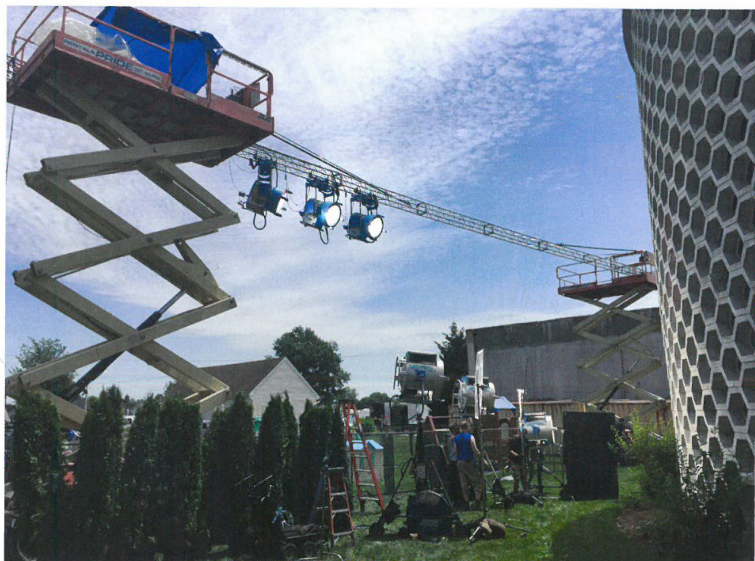
Top: Shot by Morano, the fourth episode begins with an R&B number that transitions — without cutting — into a funeral scene. Middle: For the scene, Morano's crew rigged three 12Ks on a truss that was suspended between two scissor lifts placed outside the location. Bottom: Morano captures a musical sequence featuring Buddy Holly (Philip Radiotes) near the Coney Island Cyclone roller coaster.
